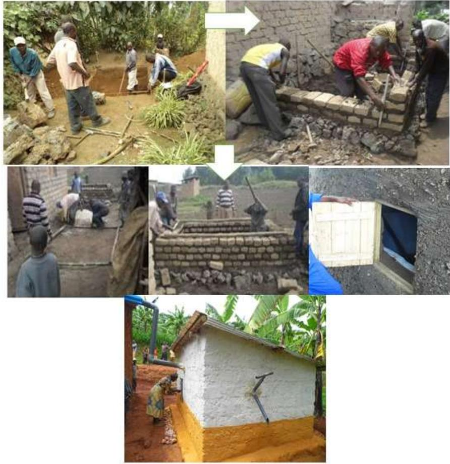
**Picture 2.2:** *Semi underground tank construction process*
