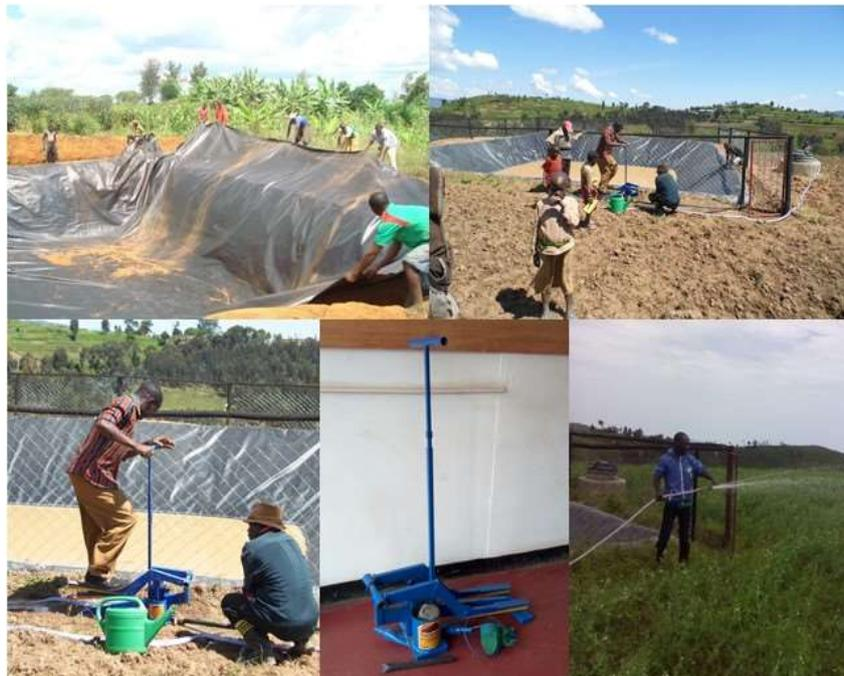
**Picture 2.3:** *Runoff water pond construction process*
