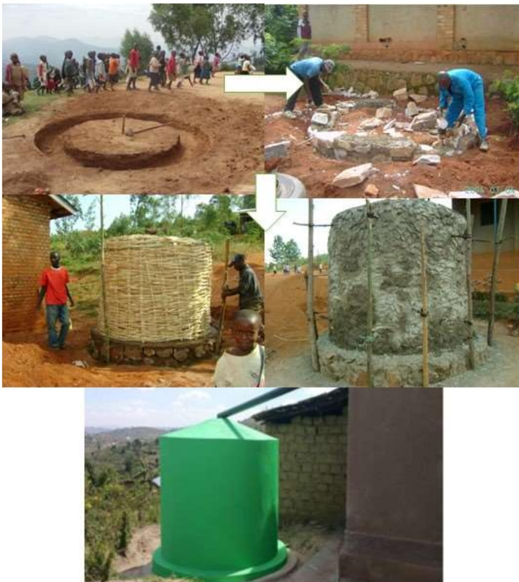
**Picture 2.1:** *Bamboo tank construction process*
