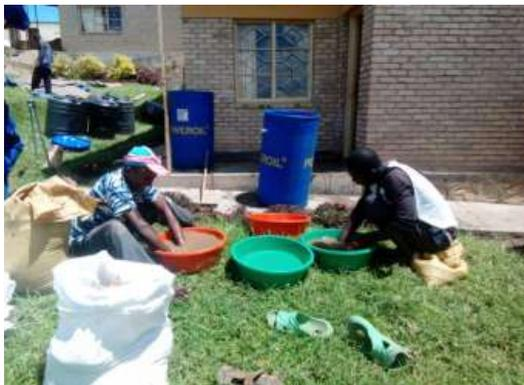
Sand being washed before use; the sand must be washed until you get clear water
