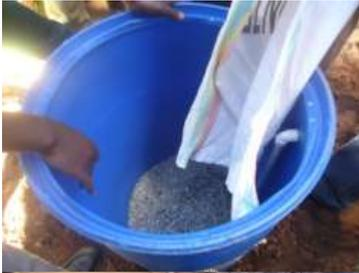
Filling the container with sand and gravel according to the sand sizes
