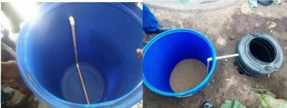
Fix the pipe system in the container and connect it to the receiving container both installed in a suitable/chosen place.
